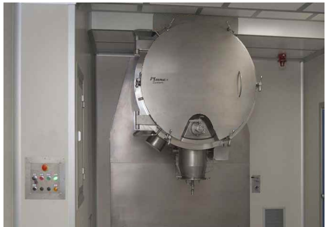
Clean room installation
