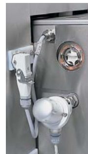
Recirculating pump station
